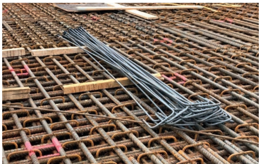
Dextra Pressed Connection headed bars being used as shear links for the main nuclear island raft
